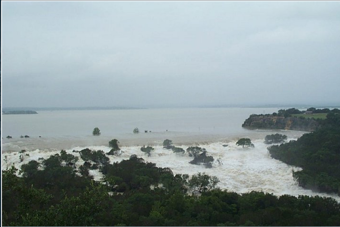
Canyon Lake spillway, Guadalupe River, Texas 70,000 ft 3 (2000 m 3 ) per second of water July 2002
