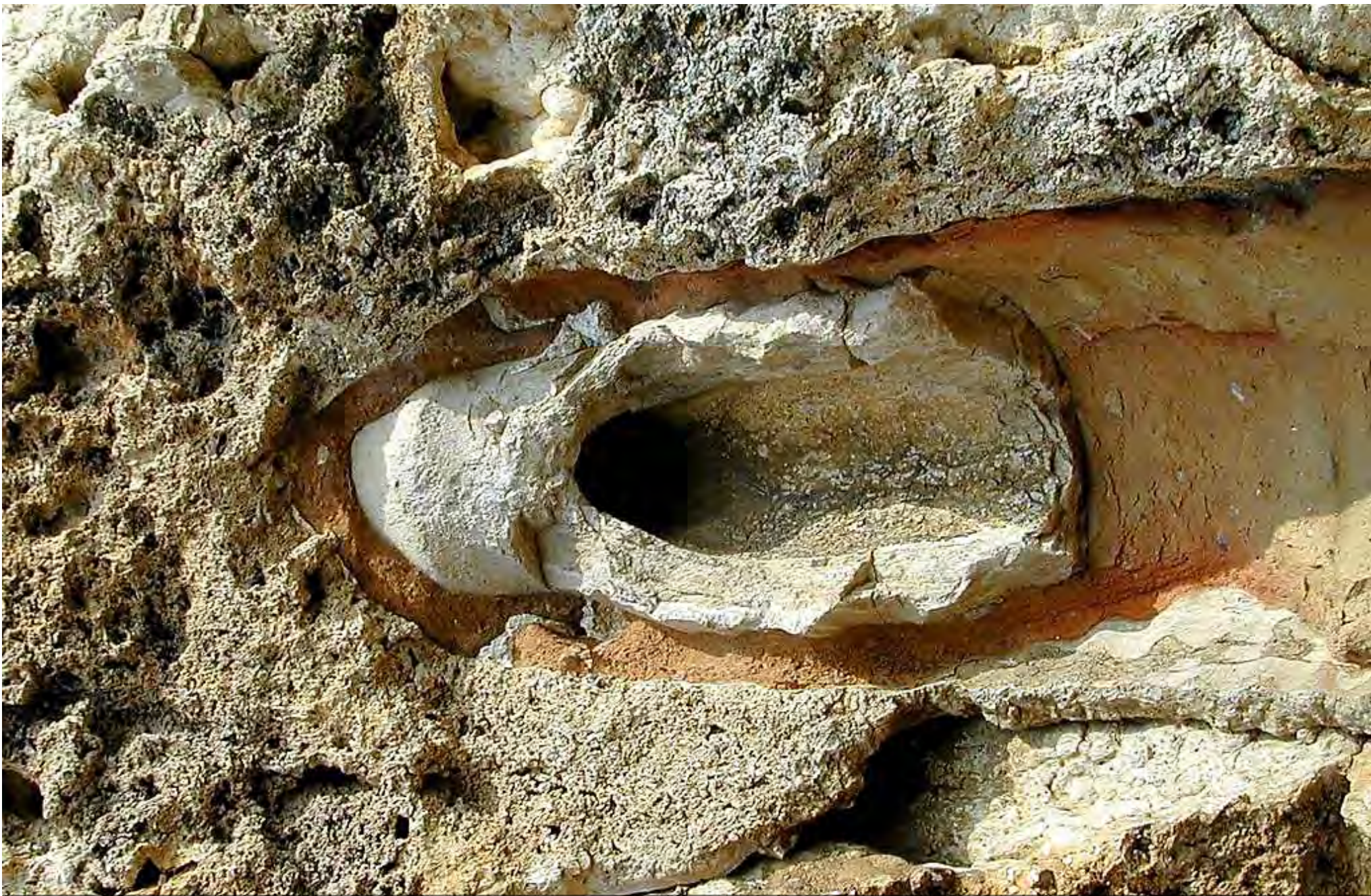
Laodicea pipe with calcium
